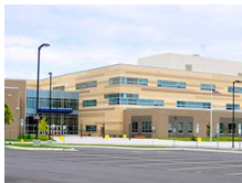
Severna Park High School building which replaced the original building.
